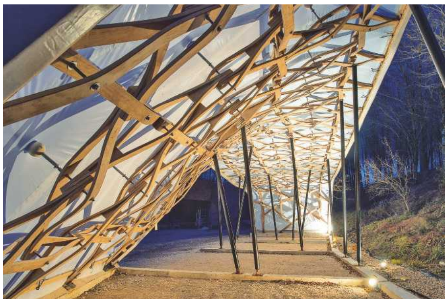
The complex structure is ready to store timber for future building projects
